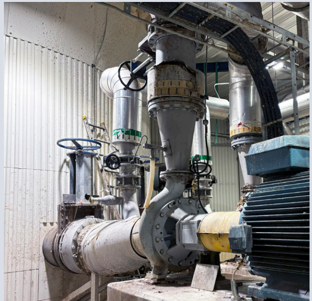
DN 600 / 24" Stafsjö MV pulp stock tower installation.
